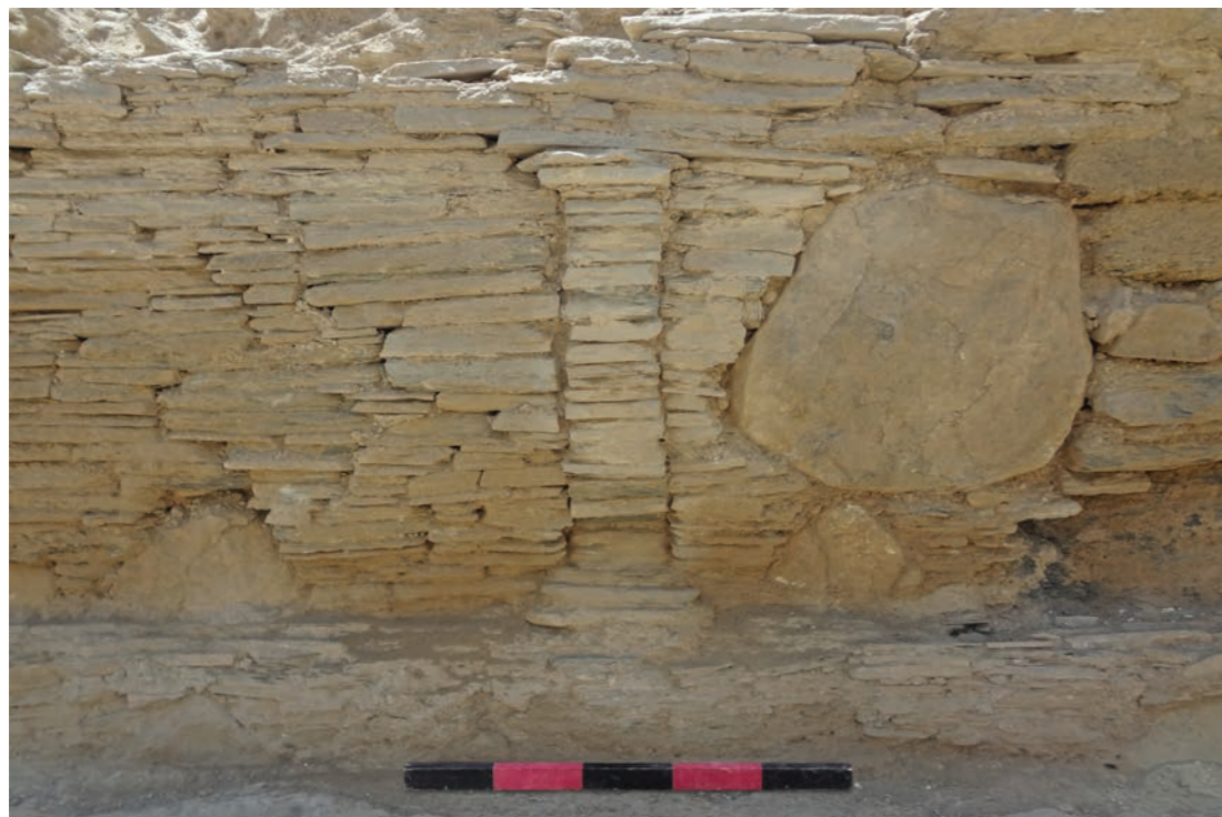
Detail of north elevation of the excavated plinth, prior to stabilization 2017
