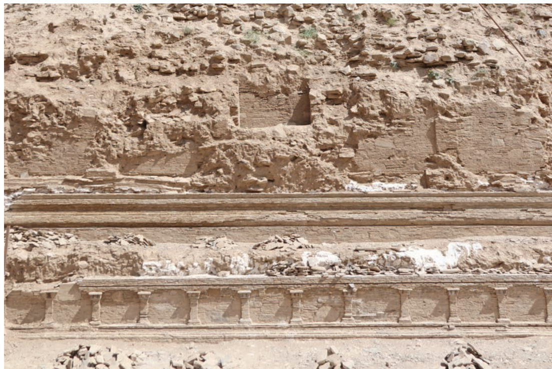
Excavated plinth and platform masonry on south elevation, with niche 2017
