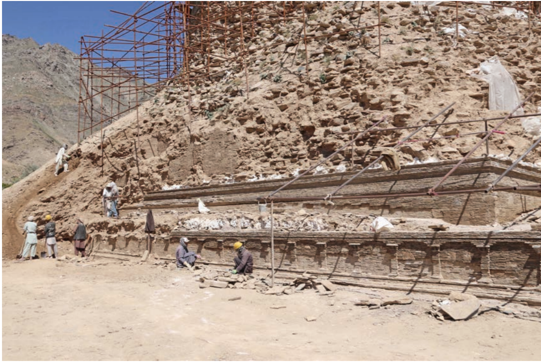
Initial stabilization of the south side of the plinth and platform 2017
