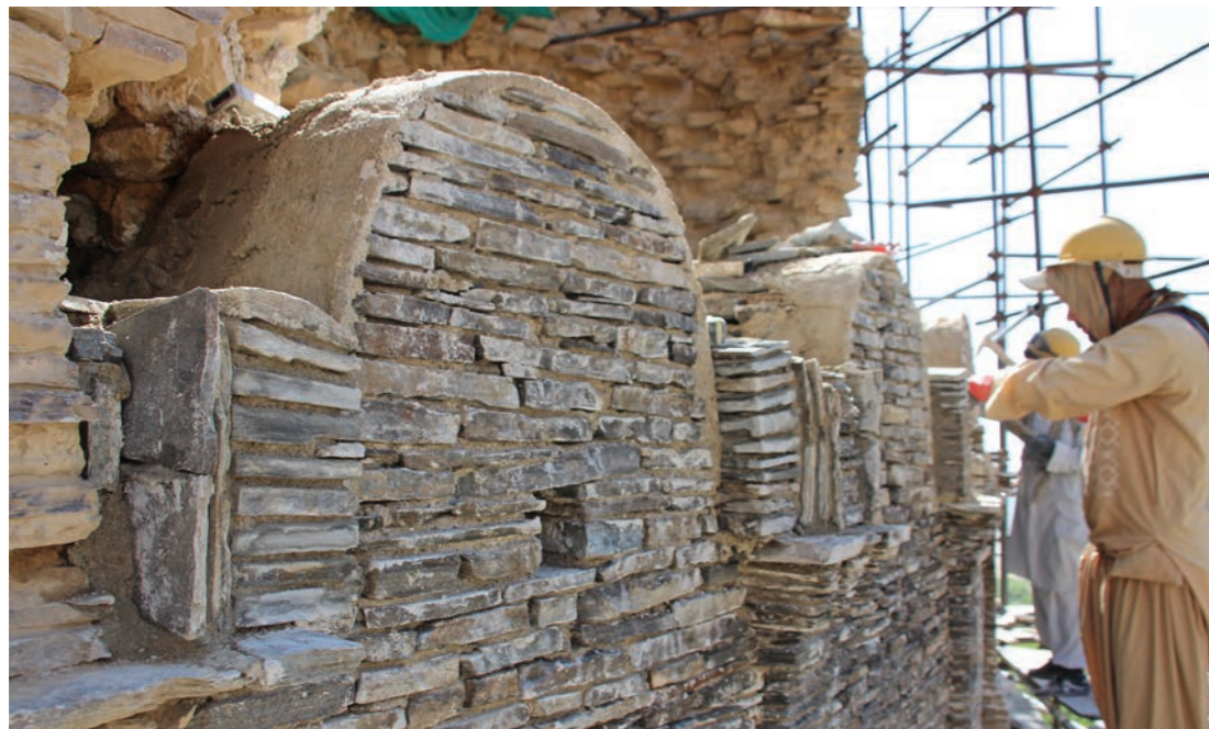
Reconstruction of collapsed section of the arcade around the drum 2017
