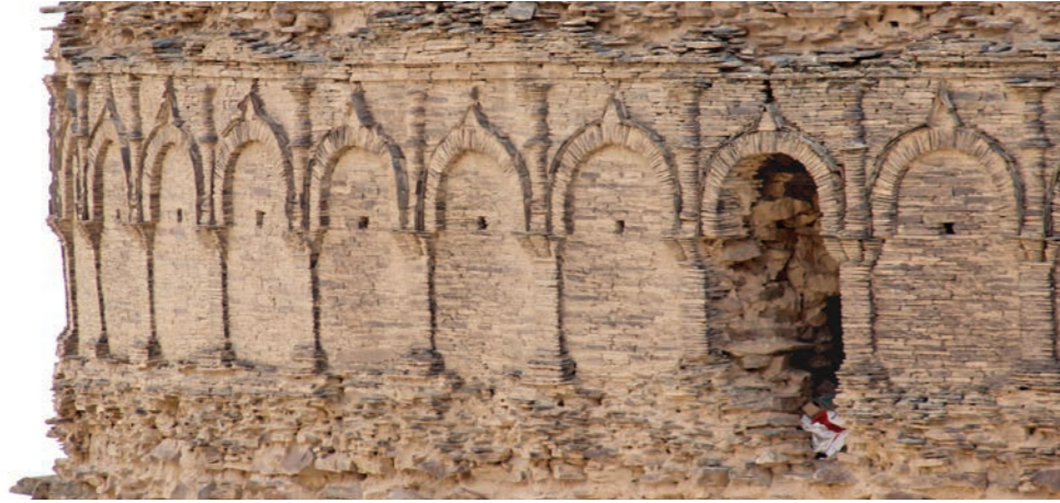
Cavity on the north side of the arcade around the drum 2016
