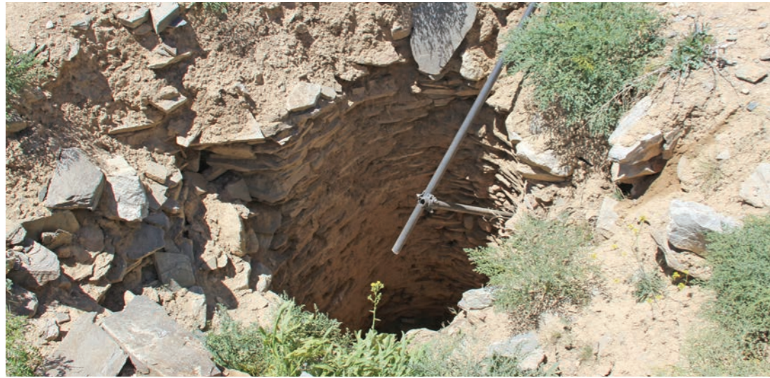
Cavity in the apex of the stupa dome, prior to capping 2017
