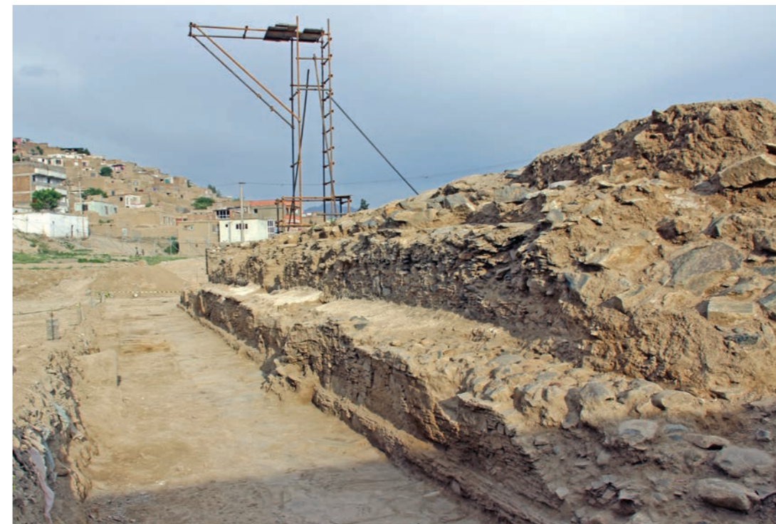
Plinth (center) along the north side in front of platform masonry. The tower in the background was constructed for photographic surveys 2017
