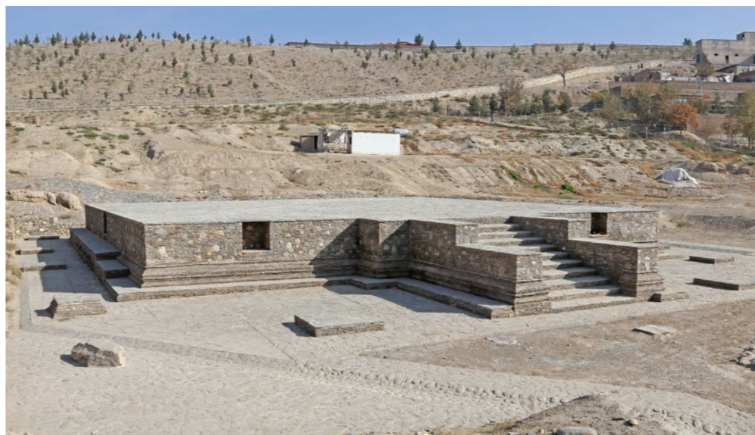
Stupa platform at Tepe Maranjan after conservation, from the south 2018
