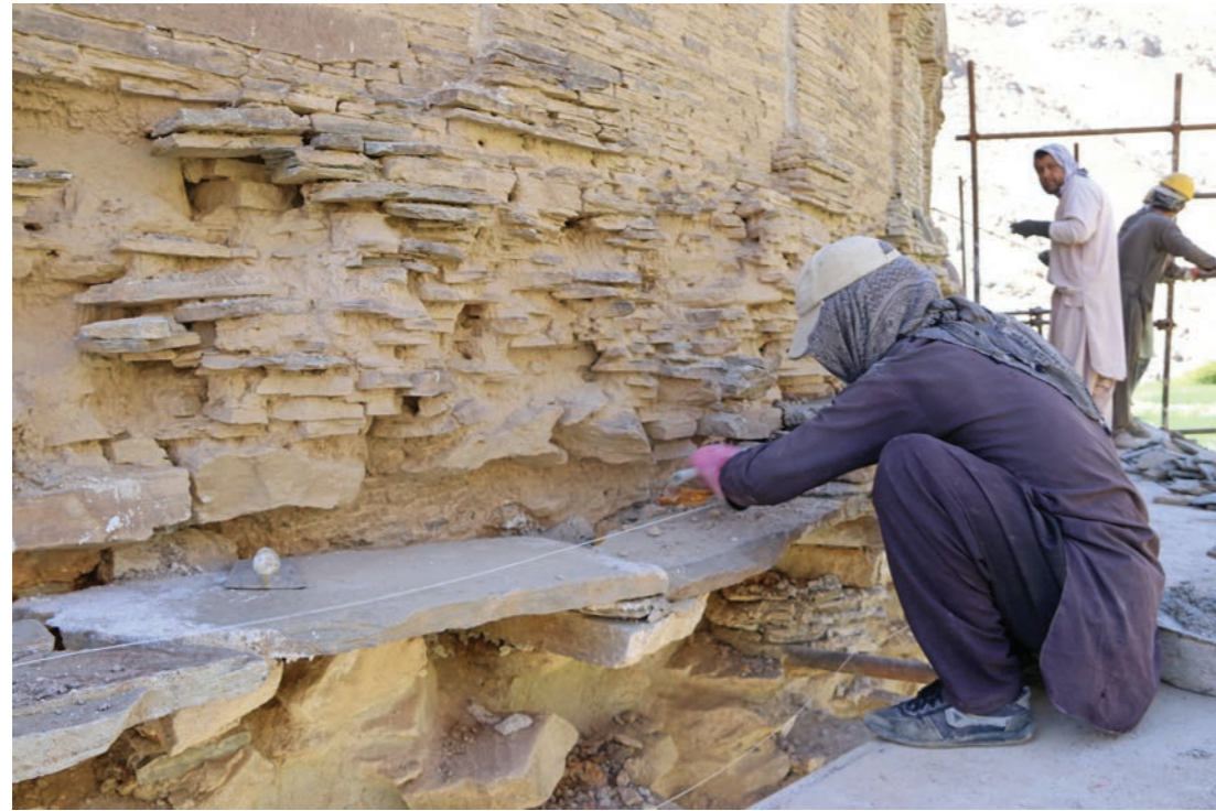
Cantilever for lower string course under construction 2018
