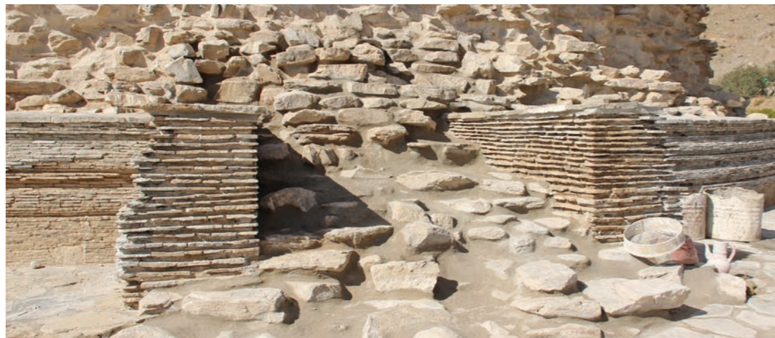
Upper stair on the east side at Topdara, after stabilization 2019
