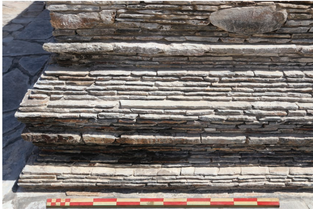
Detail of restored string-course at base of stupa platform at Tepe Maranjan
