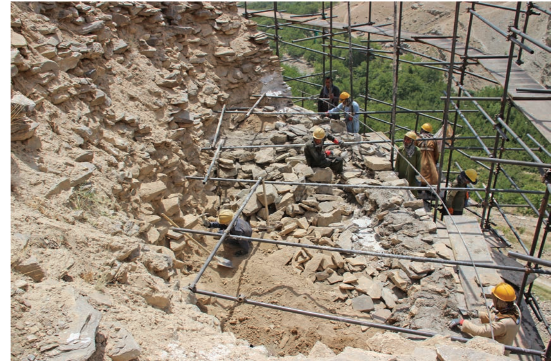
Laying masonry infill during repairs to the stupa dome 2017
