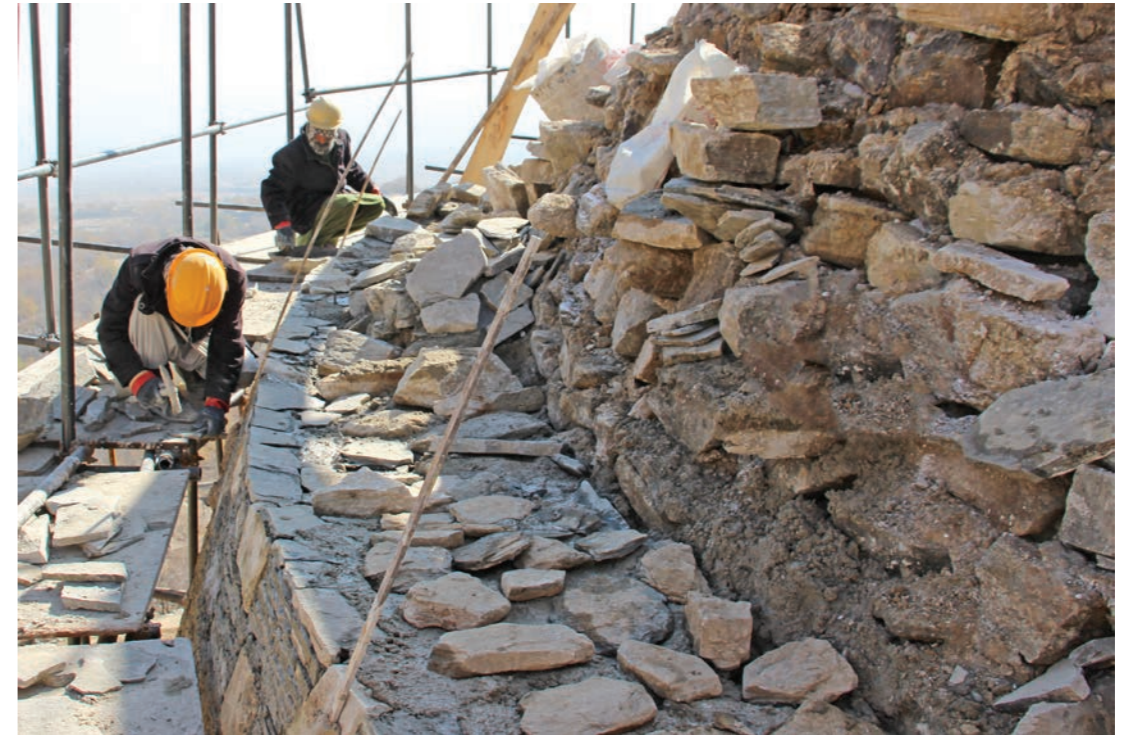
Laying masonry around the outer edge of the dome 2017
