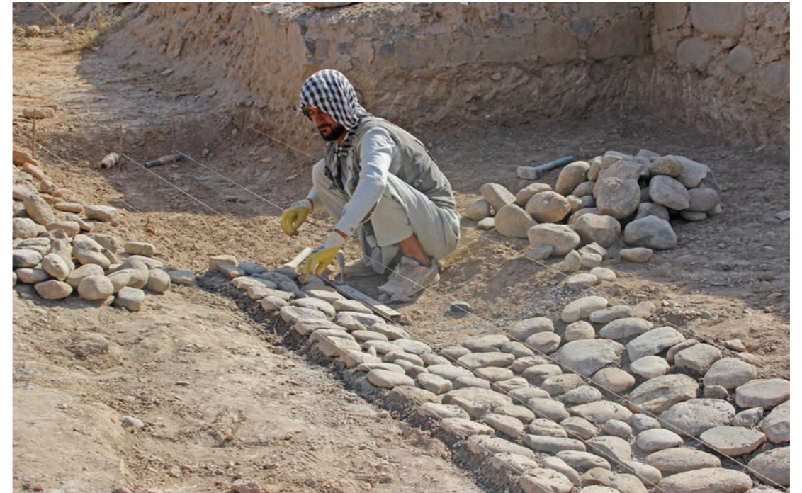
Construction of surface drain to the west of the platform 2018
