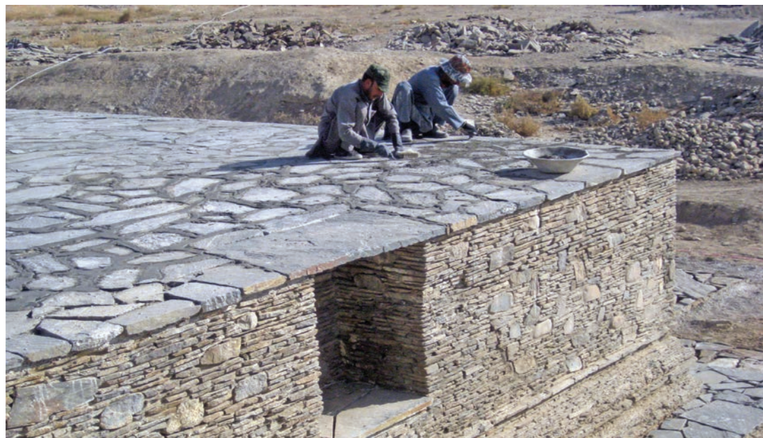
Laying stone paving on the platform surface 2018
