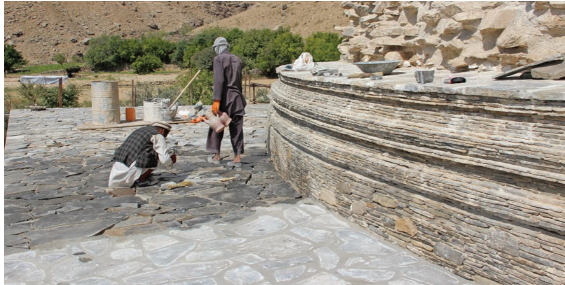
Paving stone paving over the surface of the platform and ambulatory 2019
