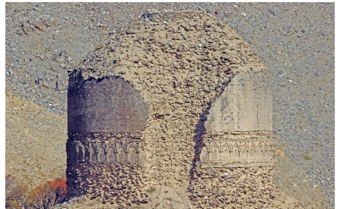
Collapsed section of stupa drum and dome to south 2016
