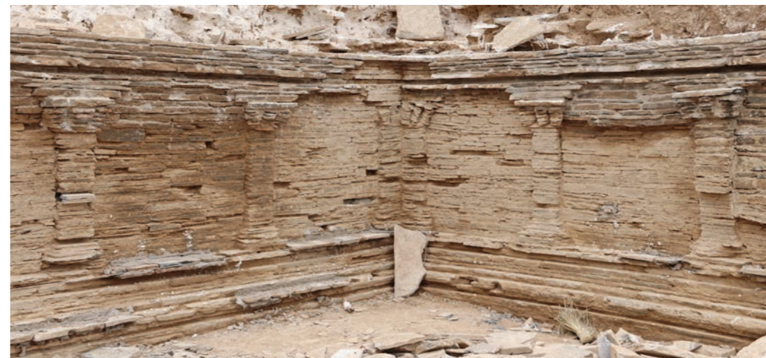
Detail of original masonry (lower part) and infill above on plinth 2017
