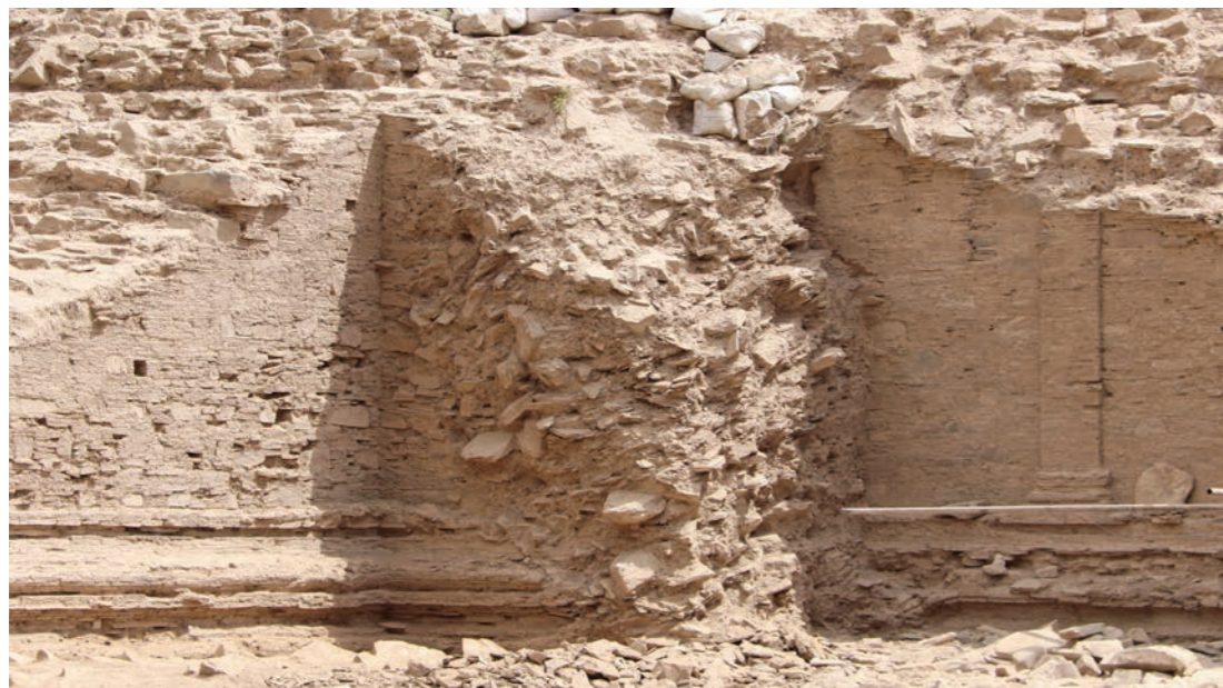
Buttress on west side of stupa platform at Topdara, before stabilisation 2018
